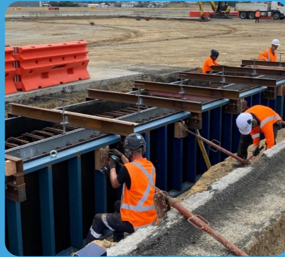
Installation of new stormwater management system
