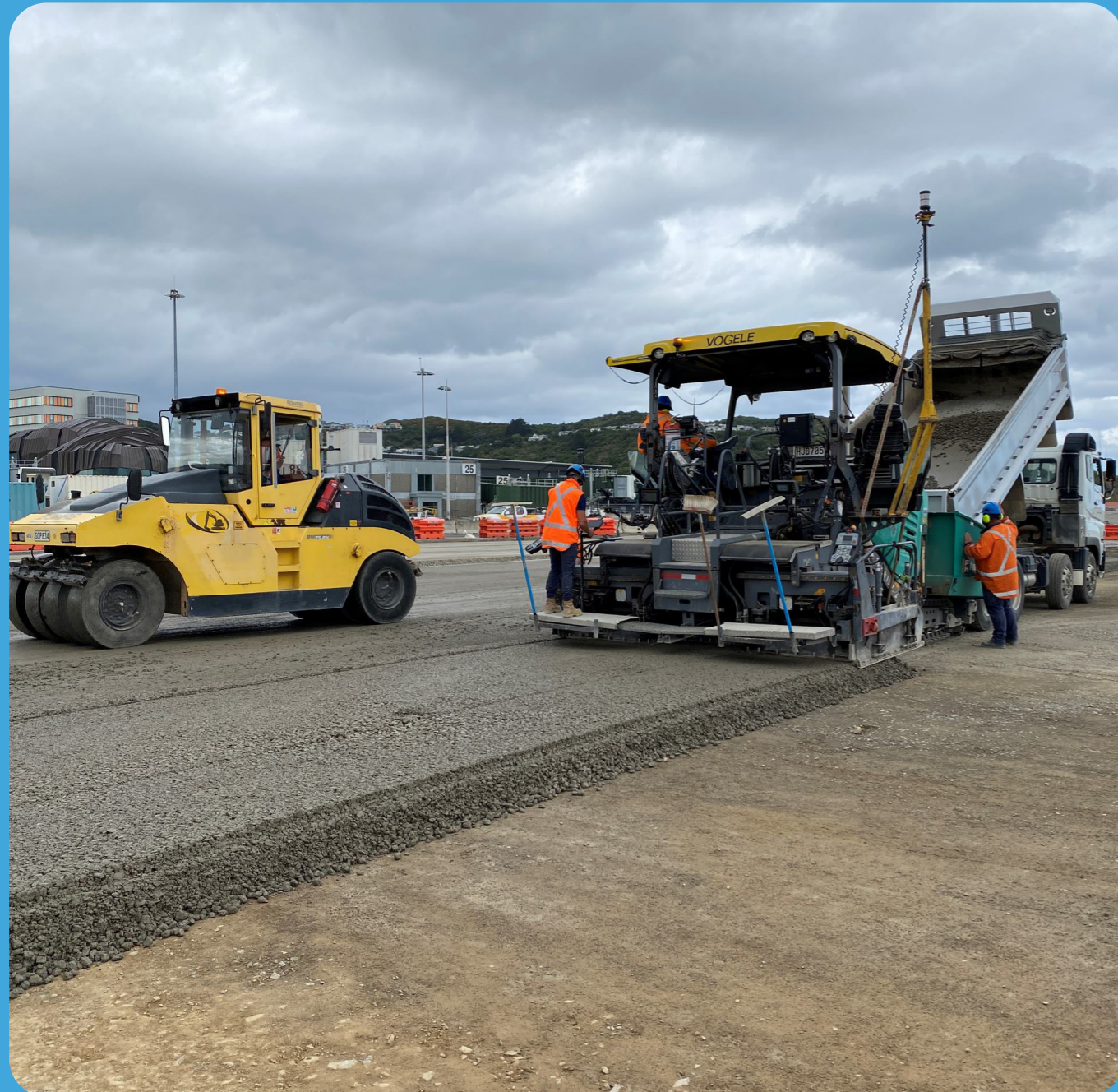
Reconstruction on Taxiway Bravo
