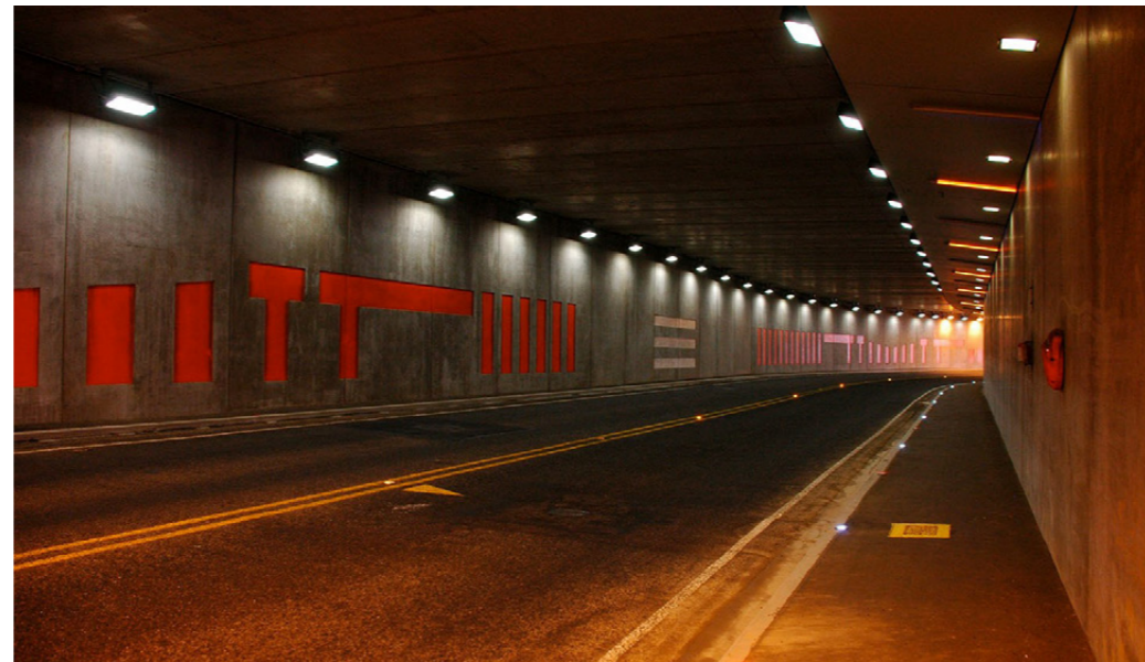
CONCRETE TILT SLAB WITH BAS-RELIEF PATTERNS - WELLINGTON AIRPORT SOUTH RESA TUNNEL
