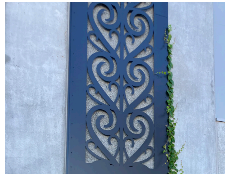
CONCRETE TILT SLAB WITH BAS-RELIEF PATTERNS - WELLINGTON AIRPORT SOUTH RESA TUNNEL
